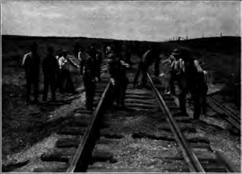
THE FINISHING TOUCHES TO THE TRACK
